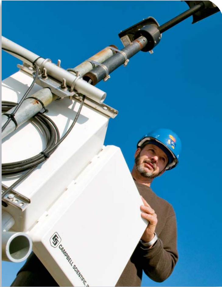
Dan DePardo, ITTC RF electronics engineer, checks an antenna on the roof of Nichols Hall.
